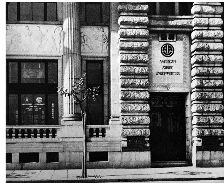
17 The Bund The North China Daily News Building became AAU headquarters in 1927.
